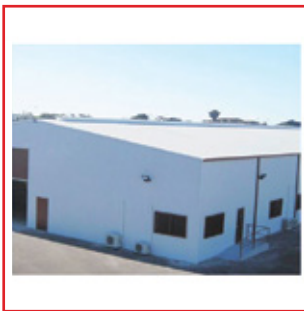
Prefab Warehouse & Workshop
